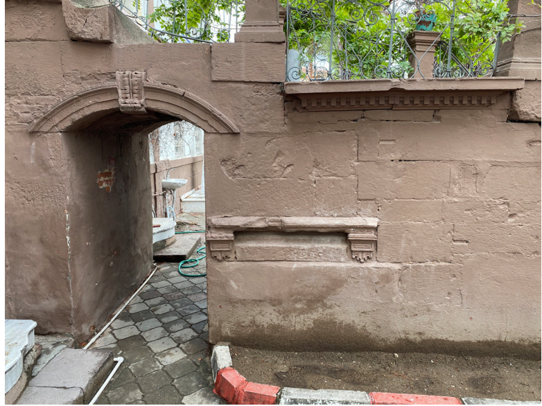
Figure 5. Çamdibi Village School, foundation of the stairs leading to the main entrance, showing reused blocks, pedestals and various ornamental elements; also visible are the adjacent marble steps before the side entrances. Source: Hasan Sercan Sağlam, 2025.
